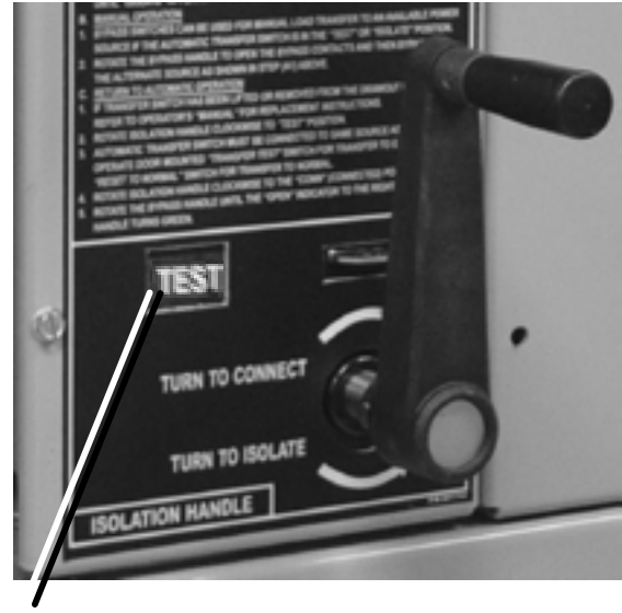
Figure 3-17. Isolation Handle turned to TEST .
