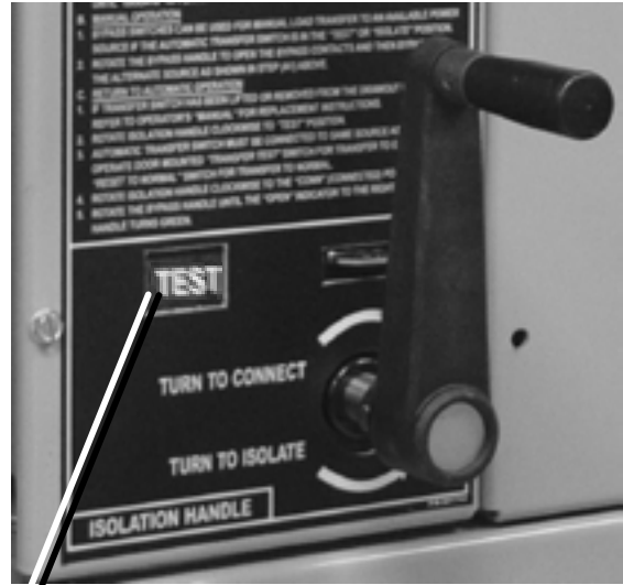
Figure 3-17. Isolation Handle turned to TEST .
